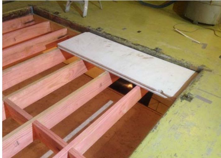
Figure 1: Installing the Rockcote panels on the timber joists
