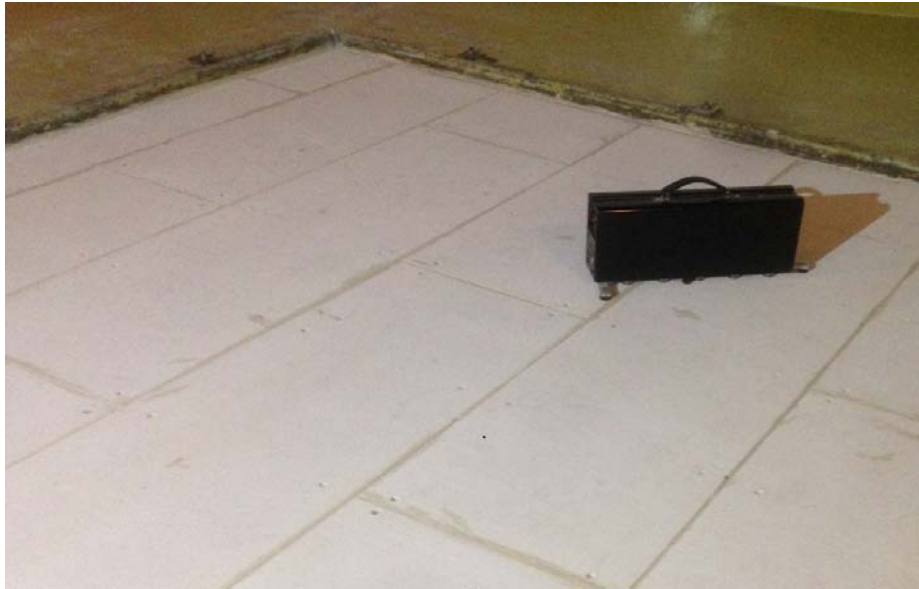
Figure 3: One of the tapping machine positions on the completed floor
