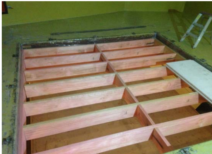
Figure 2: Floor joists framing showing the central nogs.
