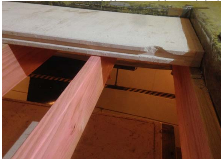
Figure 1: Rockcote panels sitting on timber joist floor structure
