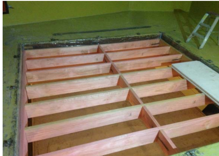
Figure 2: Floor structure installed in floor test cavity
